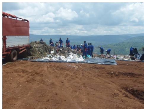
The first day of waste reception at Nduba tentative landfill
