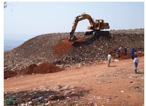
First soil coverage at Nyanza landfill (July 2010)
