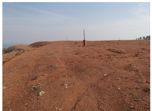
Nyanza landfill after its final closure by following the Fukuoka Method (August 2013)
