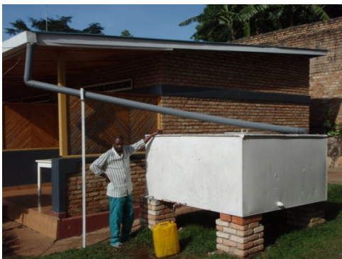
Original rain water collection tank found in Butare
