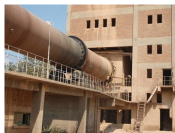
Facility at a cement factory in Rwanda where removed asbestos cement roofs could be incinerated properly
